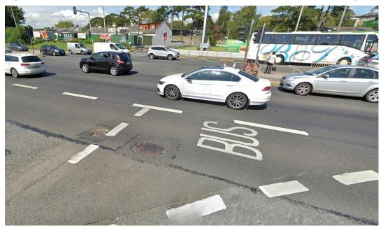
Figure 7-7 Good Road Pavement Condition on Chapelizod bypass, Palmerstown – (but with some damage around utility chamber covers) ©2020 Google Maps
